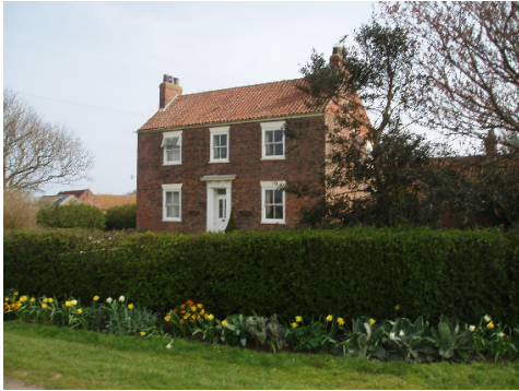
The Grange – Main Street
